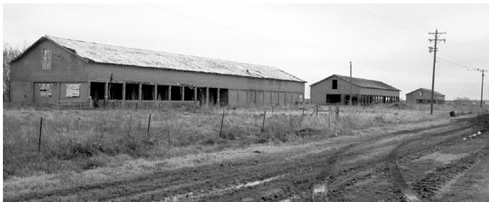
Figure 10. Central State Farm Camp No. 1 Livestock Barns (Properties 72, 73, and 74), 2004, looking northeast (photograph by author).
