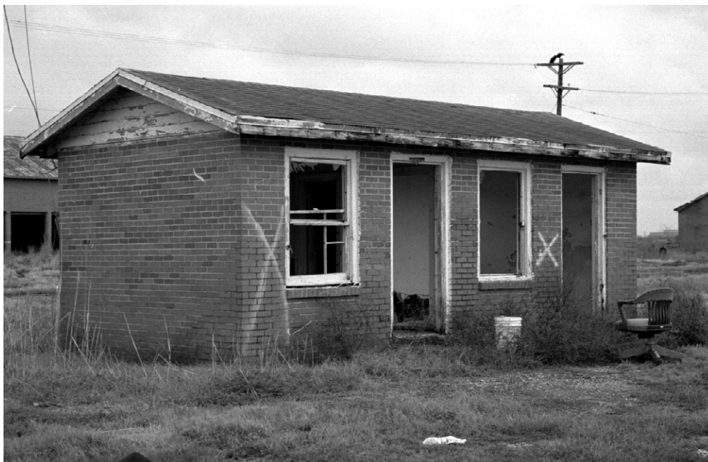
Figure 11. Central State Farm Camp No. 1 Administrative Building (Property 57), 2004, looking northeast (photograph by author).
